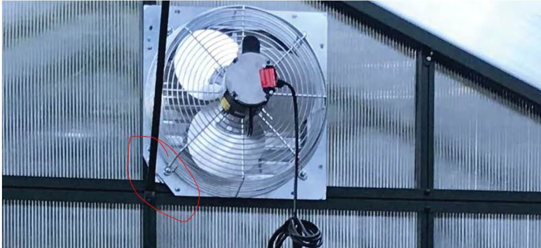
OPTION 1: Attach fan with bolts inserted into channel of PRO1456
