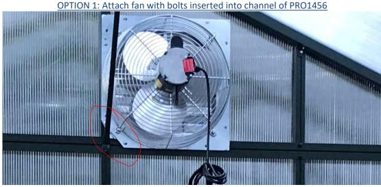
Once your panel with the cutout for the fan is in place, mount the fan on the interior of the greenhouse using bolts in the channels of the aluminum extrusions. These bolts will fit through the holes on the exhaust fan. You may need to cut the corner off due to the diagonal support beam being in the way.
