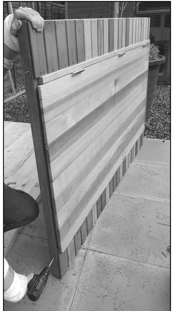
Before you can install the door section you need to fit the door handle. Slide the spindle through the lock to give you the position of the handle on the door. Fix the handle with the 3.5 x 25mm countersunk screws supplied (diagram 20). Before you offer the door up to the assembly you need to remove the transit rail from the bottom of the door panel (diagram 19).
